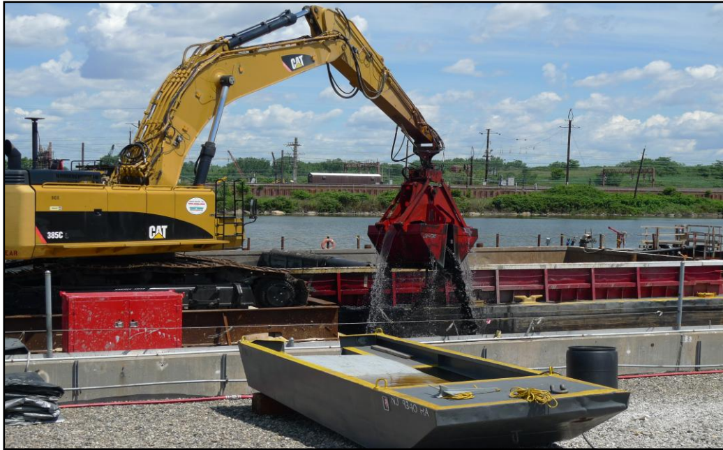
Figure 47. A mechanical dredge for sediment removal in inland waters.
